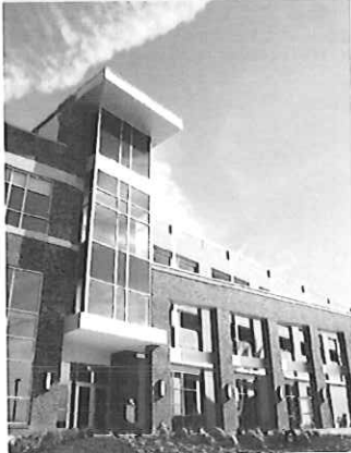
WVU Transportation Center & Garage
