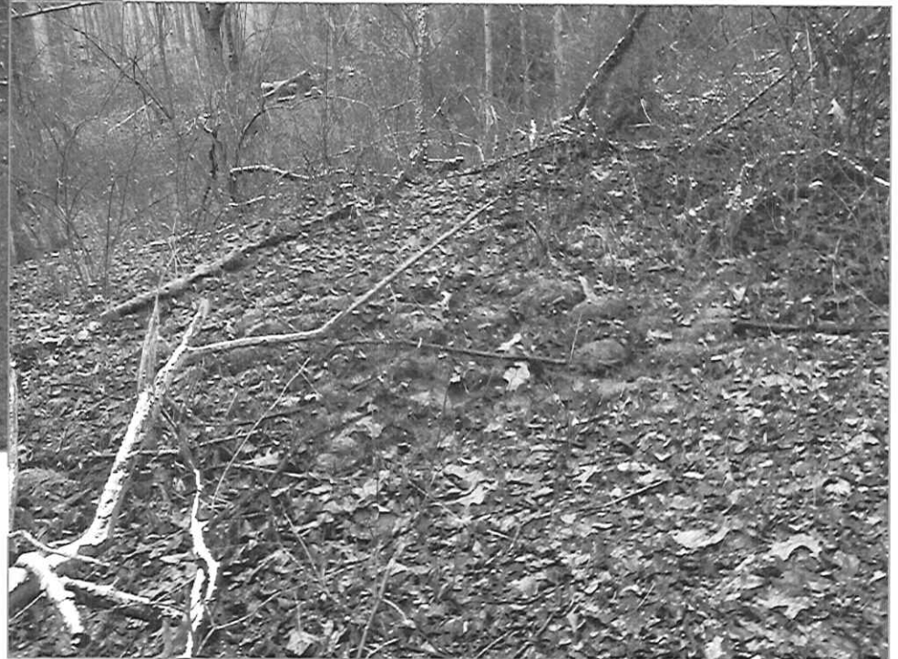
Photo "G" - Seep at Toe of Landslide
