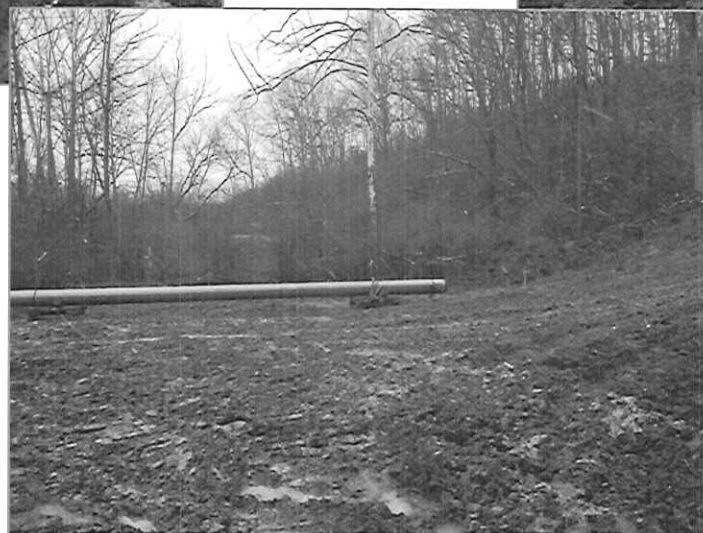
Photos "H", "I" and "J" – Current Pipeline Construction
