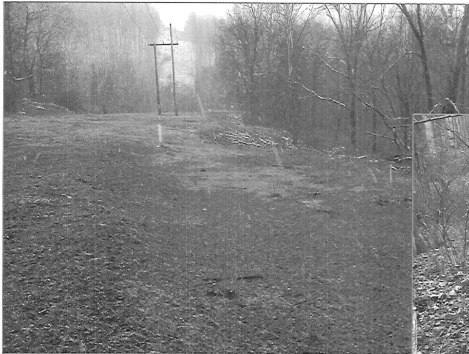
Photo "F" - Larry Frederick Landslide Area
