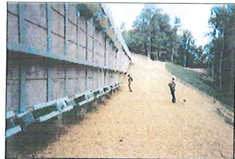
Finished wall with anchors
