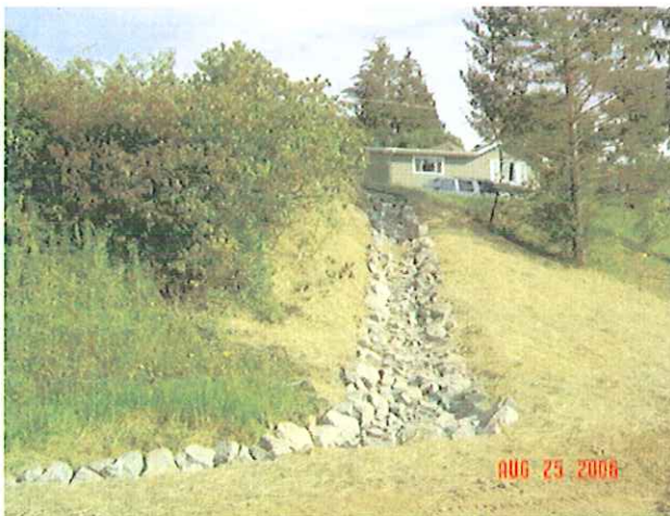
Erosion Repair – Rip Rap Armored Ditch
