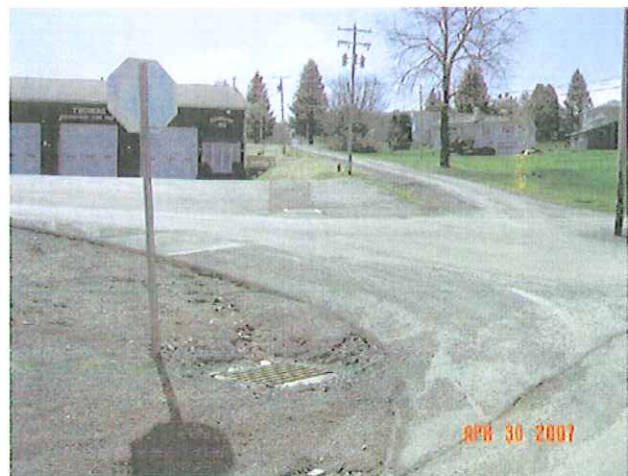
New Storm Drains and Catch Basins
