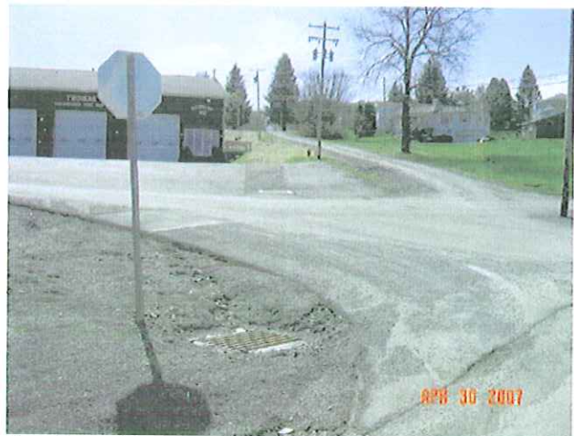
New Storm Drains and Catch Basins
