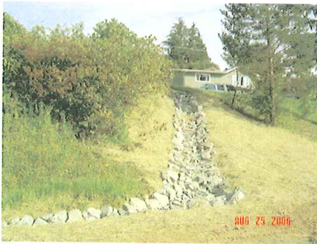
Erosion Repair – Rip Rap Armored Ditch
