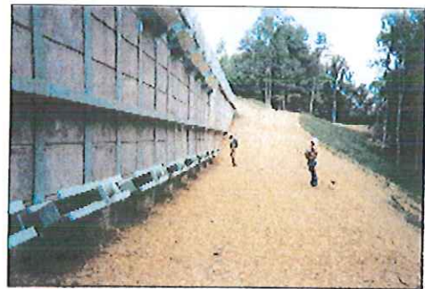
Finished wall with anchors
