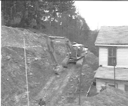
TUNNELTON (DILLSWORTH) LANDSLIDE Gabion Basket Wall Installation behind Dillsworth Residence
