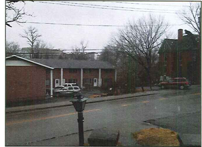
Photo G - Impacted Structure
