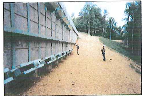
Finished wall with anchors
