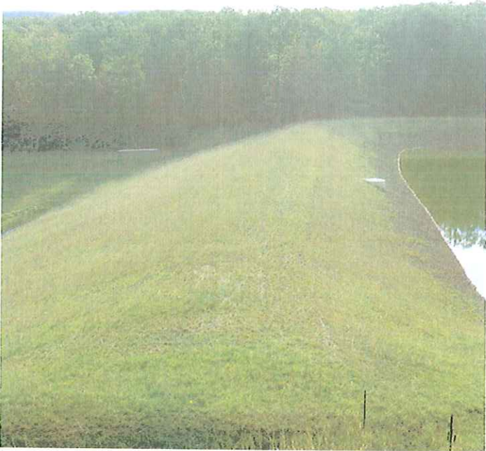
WILSON DAM MODIFICATION, HAMPSHIRE CO., WV
