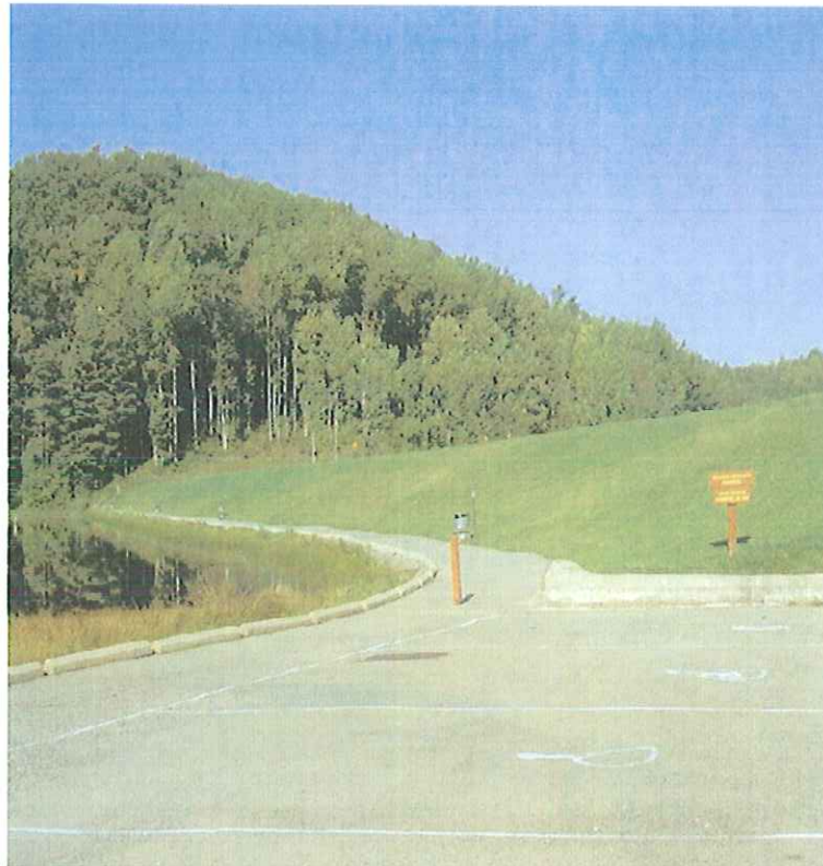
TETER CREEK DAM MODIFICATION, BARBOUR CO., WV
