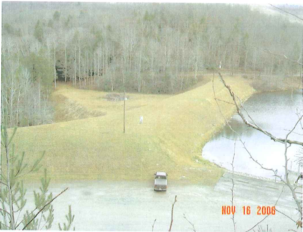
PLUM ORCHARD DAM MODIFICATION, FAYETTE CO., WV
