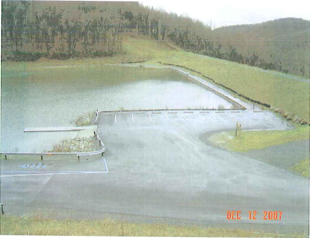
BAILEY DAM MODIFICATION, MONONGALIA CO., WV
