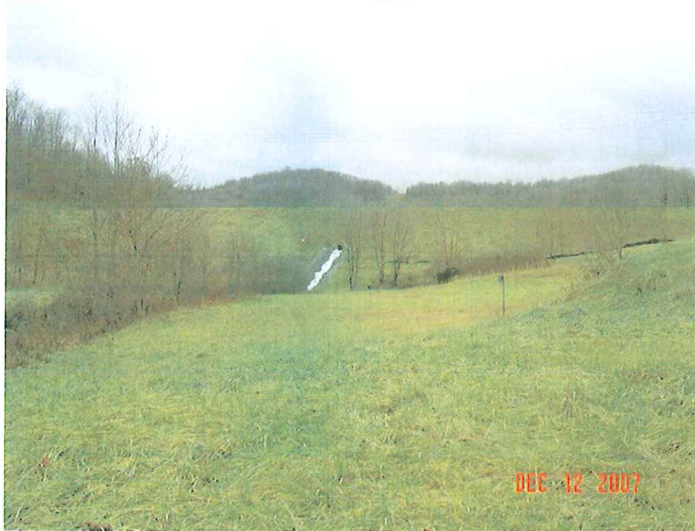
LEMLEY DAM MODIFICATION, MONONGALIA CO., WV
