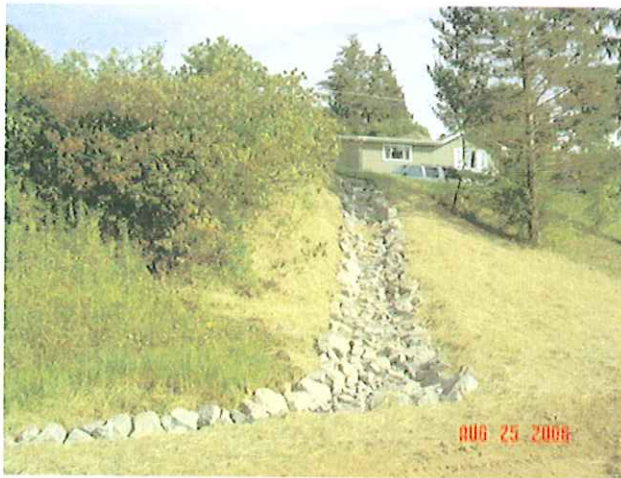
Erosion Repair – Rip Rap Armored Ditch
