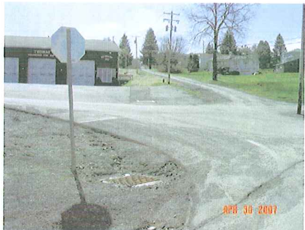
New Storm Drains and Catch Basins
