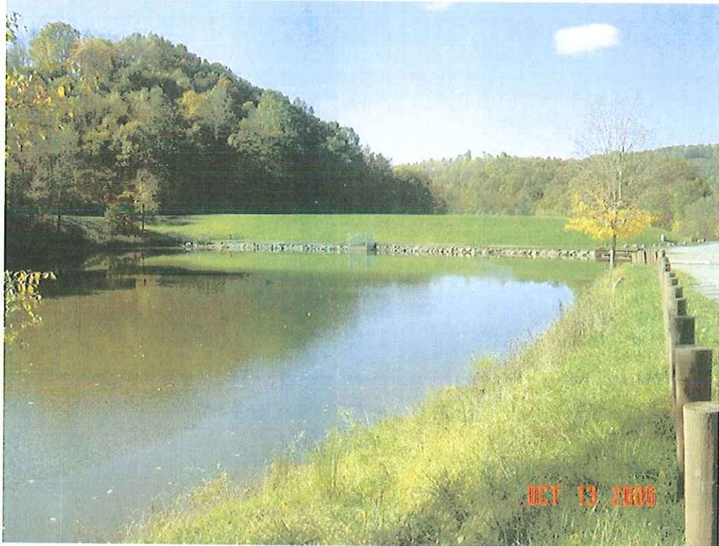
JIMMY LEWIS DAM MODIFICATION, MERCER CO., WV
