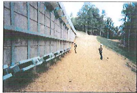
Finished wall with anchors
