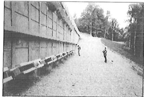
Finished wall with anchors
