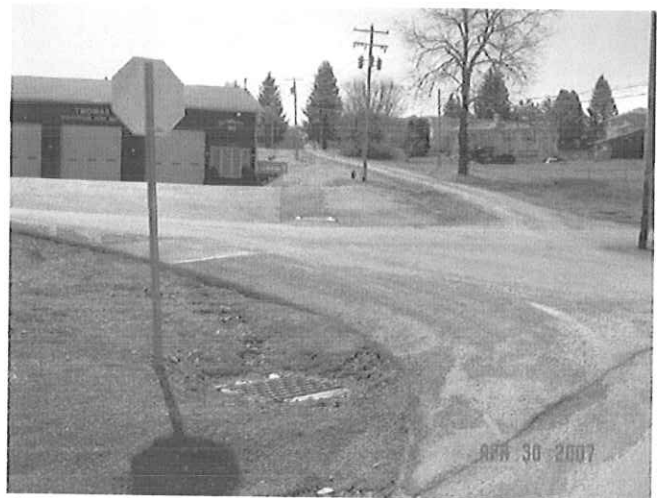
New Storm Drains and Catch Basins
