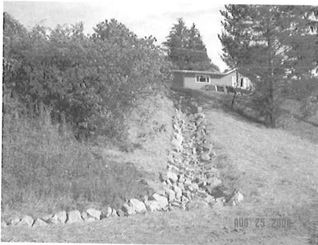
Erosion Repair – Rip Rap Armored Ditch
