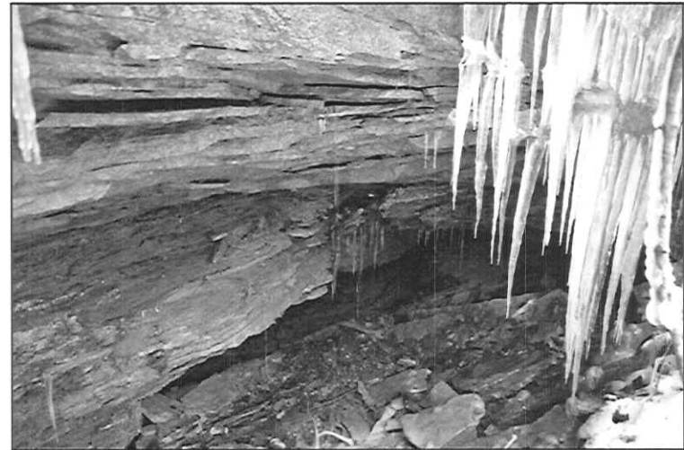
Photo B - Portal No. 3
