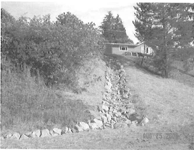
Erosion Repair – Rip Rap Armored Ditch
