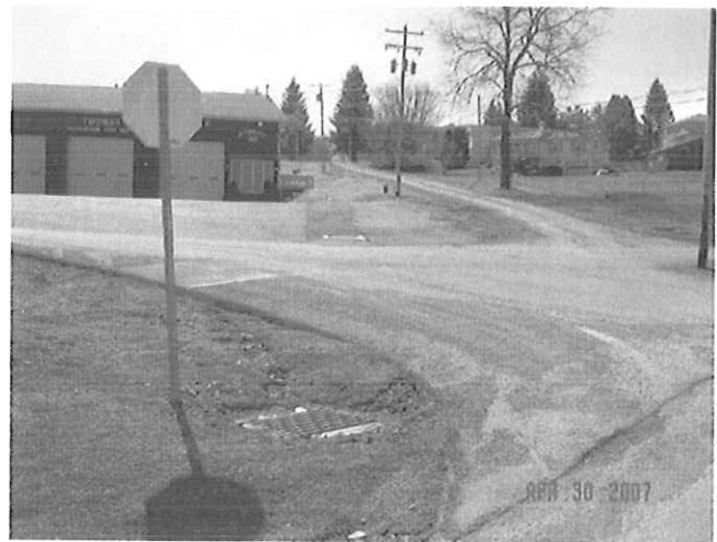
New Storm Drains and Catch Basins
