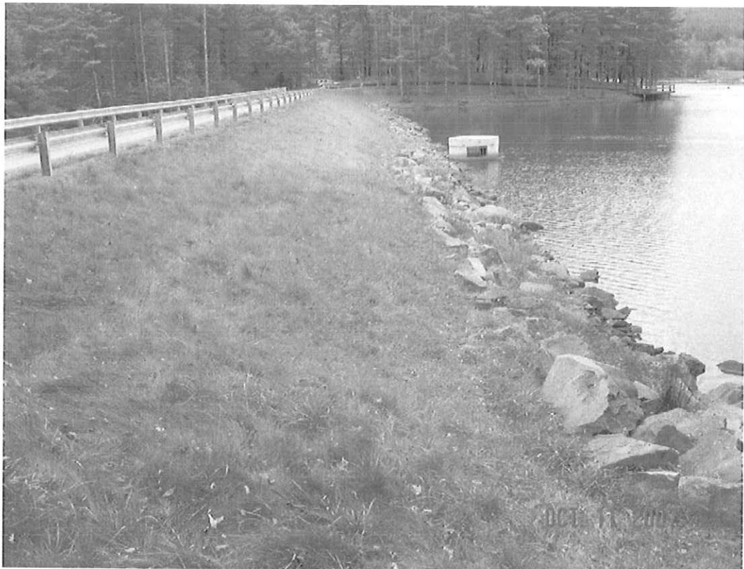
MONCOVE DAM MODIFICATION, MONROE CO., WV
