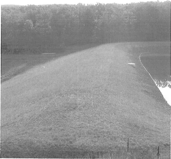
WILSON DAM MODIFICATION, HAMPSHIRE CO., WV
