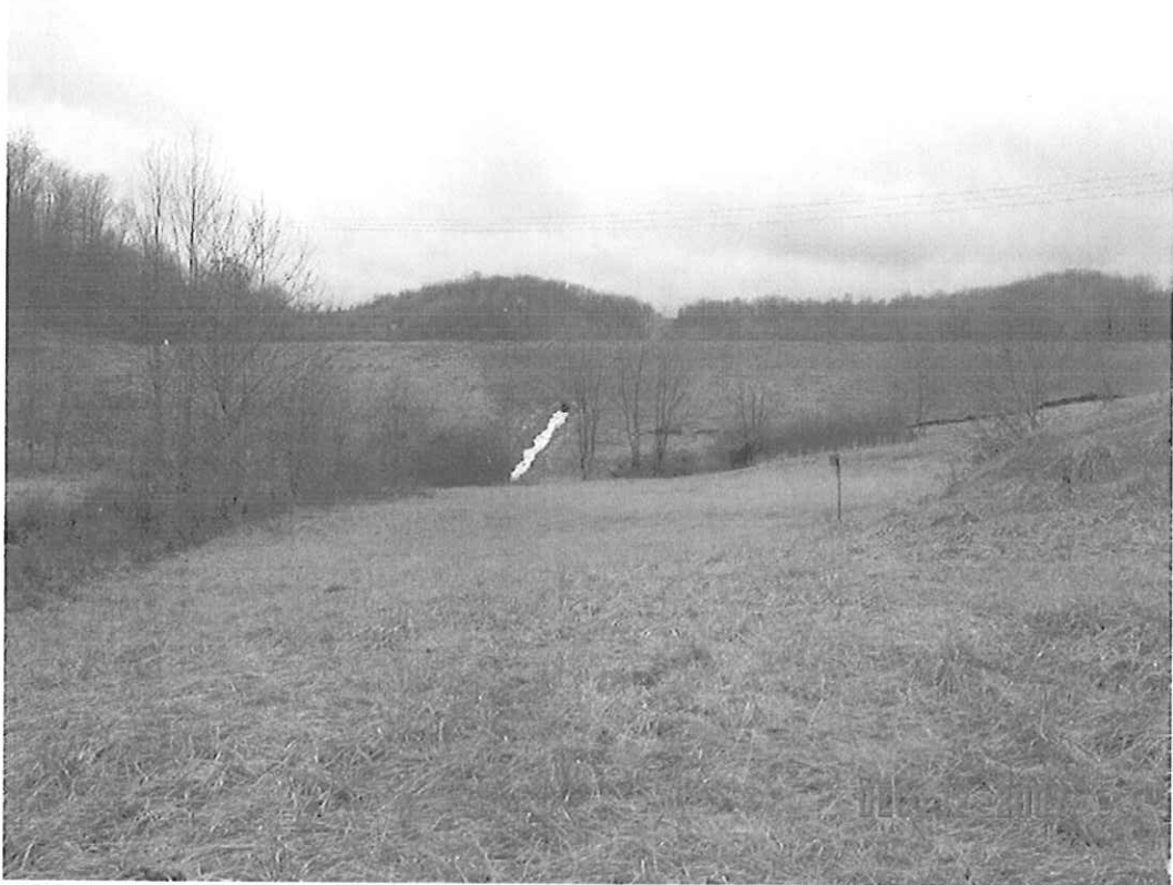
LEMLEY DAM MODIFICATION, MONONGALIA CO., WV
