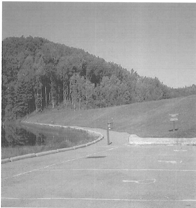
TETER CREEK DAM MODIFICATION, BARBOUR CO., WV
