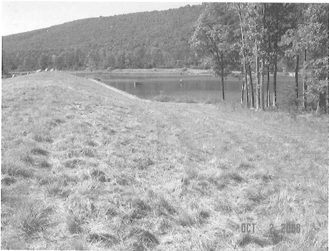
WARDEN LAKE DAM MODIFICATION, HARDY CO., WV
