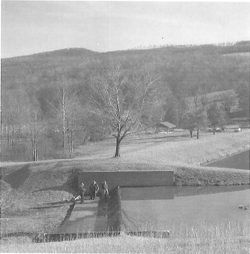
BELINGTON DAM MODIFICATION, BELINGTON, WV
