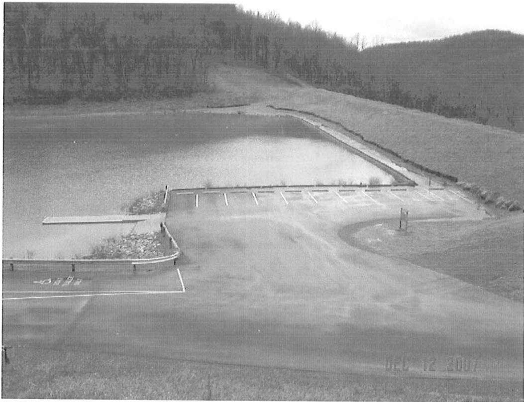
BAILEY DAM MODIFICATION, MONONGALIA CO., WV
