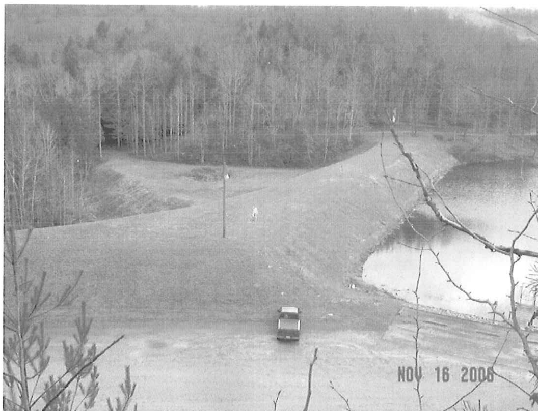
PLUM ORCHARD DAM MODIFICATION, FAYETTE CO., WV
