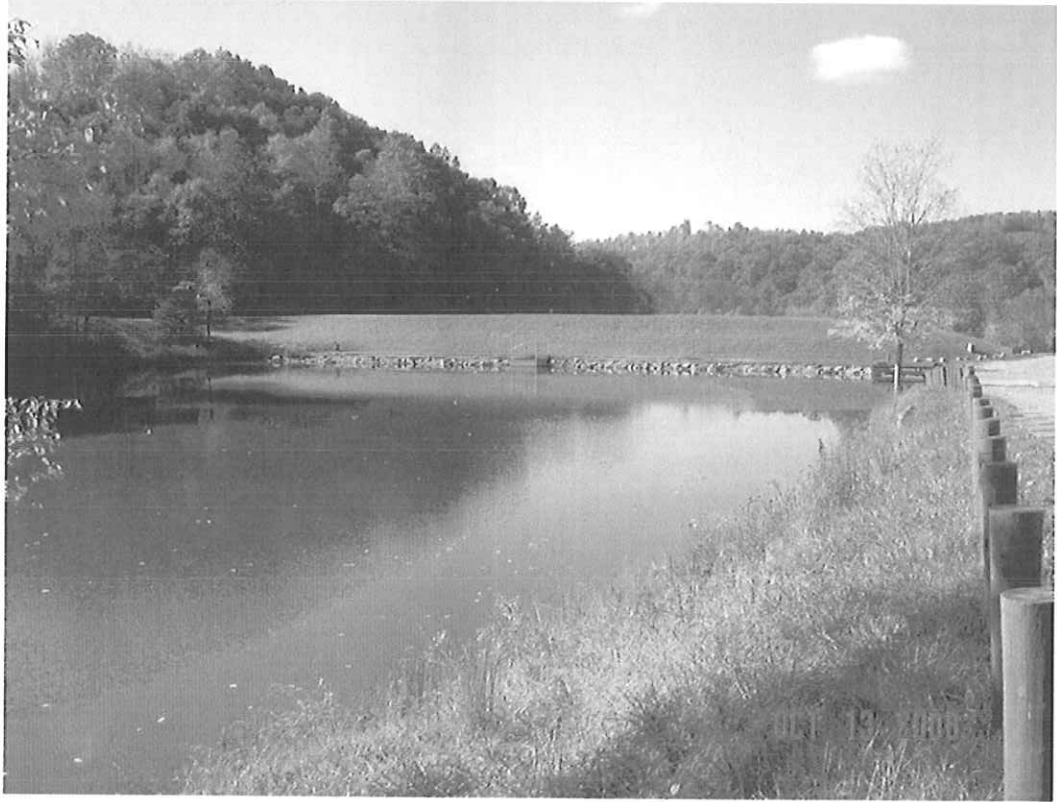
JIMMY LEWIS DAM MODIFICATION, MERCER CO., WV
