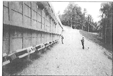
Finished wall with anchors
