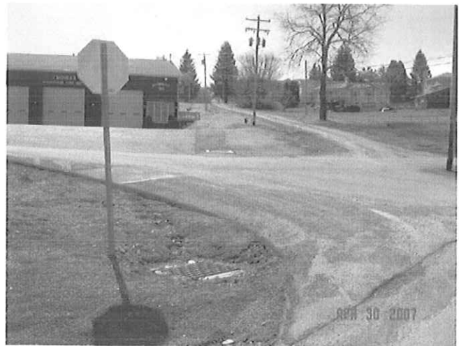
New Storm Drains and Catch Basins
