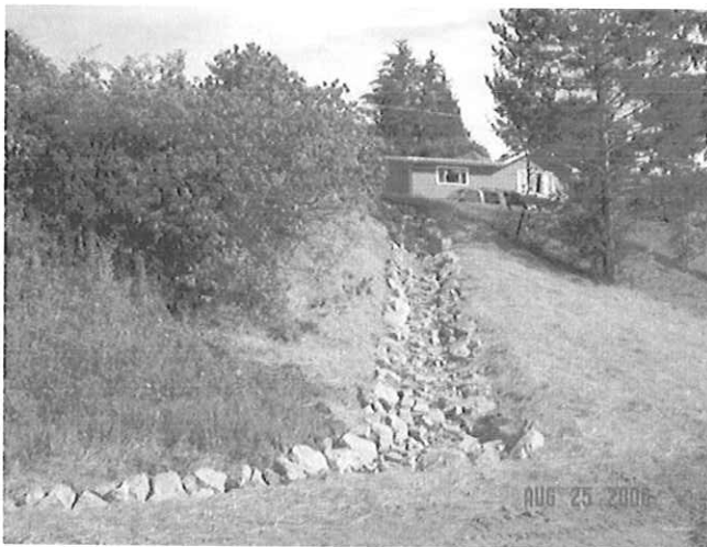
Erosion Repair – Rip Rap Armored Ditch
