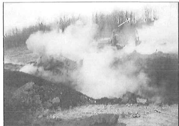
Jamison Burning Refuse Reclamation Project
