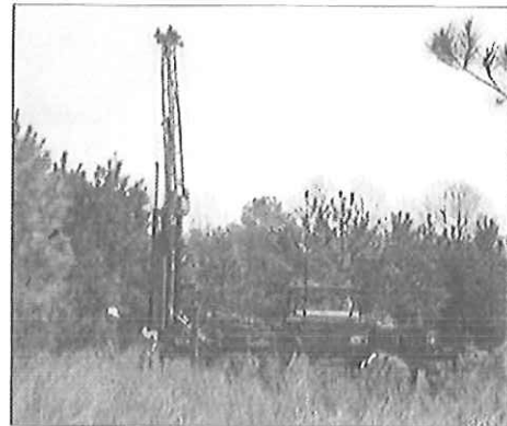
CTL's ATV can drill in rough terrain
