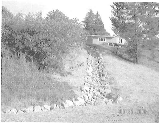
Erosion Repair – Rip Rap Armored Ditch
