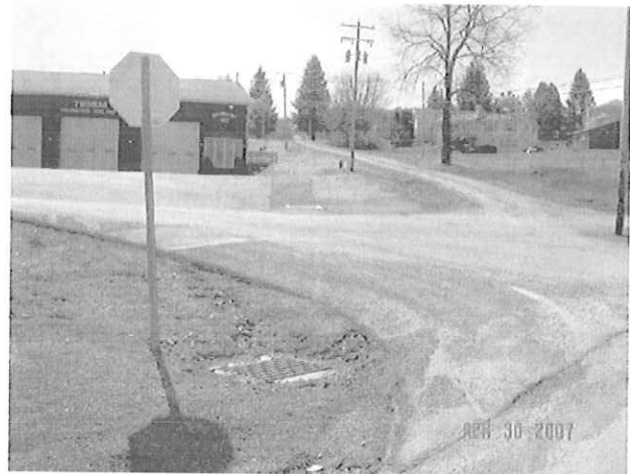
New Storm Drains and Catch Basins
