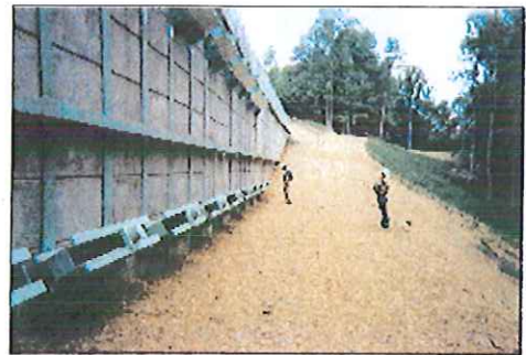
Finished wall with anchors
