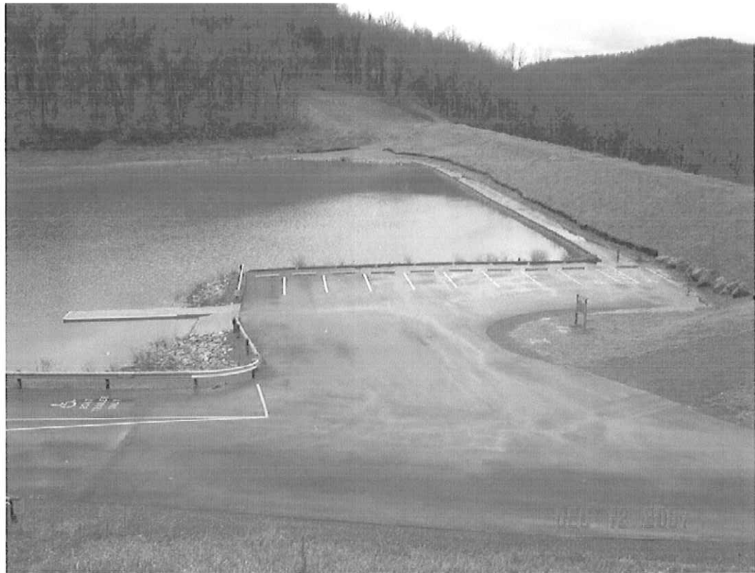
BAILEY DAM MODIFICATION, MONONGALIA CO., WV
