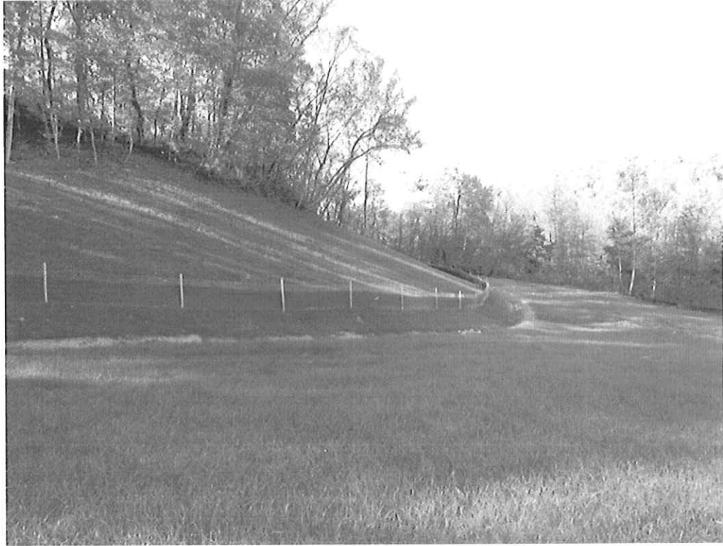
Prospect Valley Highwall #4 – DEP14433
