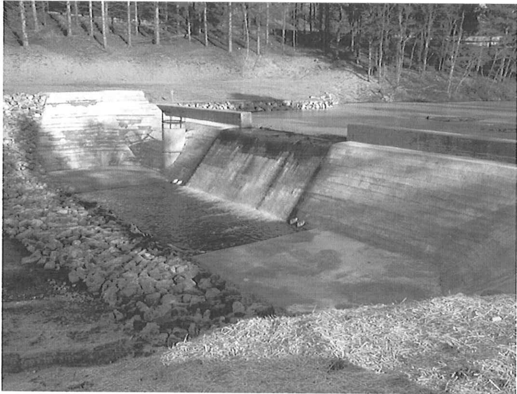
THOMAS DAM MODIFICATION, THOMAS, WV
