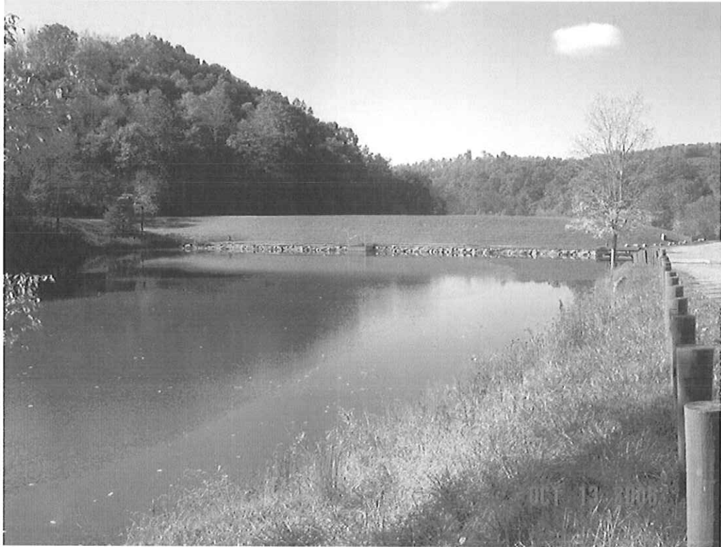
JIMMY LEWIS DAM MODIFICATION, MERCER CO., WV
