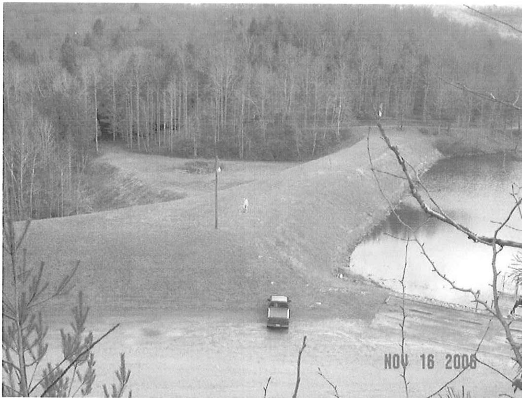
PLUM ORCHARD DAM MODIFICATION, FAYETTE CO., WV
