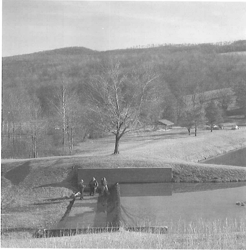
BELINGTON DAM MODIFICATION, BELINGTON, WV
