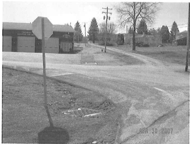
New Storm Drains and Catch Basins
