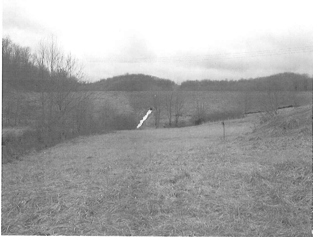
LEMLEY DAM MODIFICATION, MONONGALIA CO., WV
