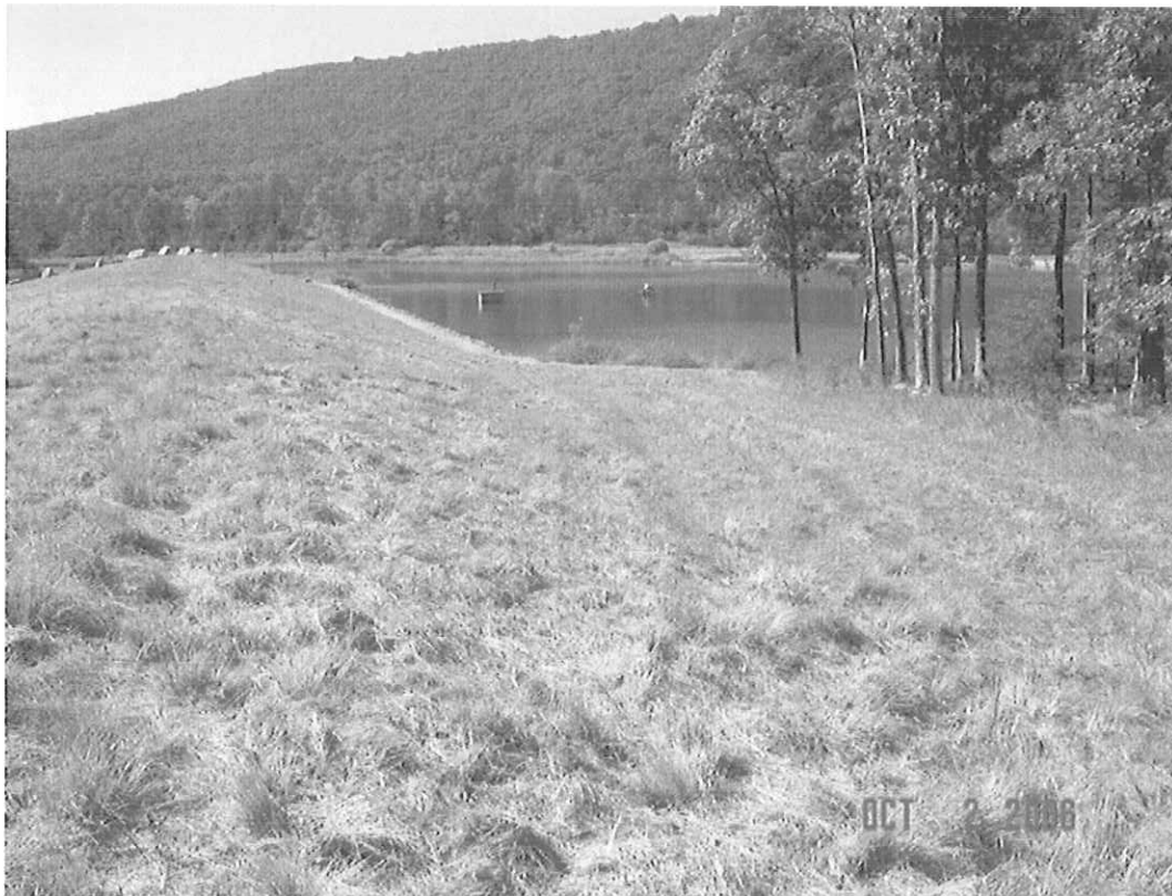
WARDEN LAKE DAM MODIFICATION, HARDY CO., WV
