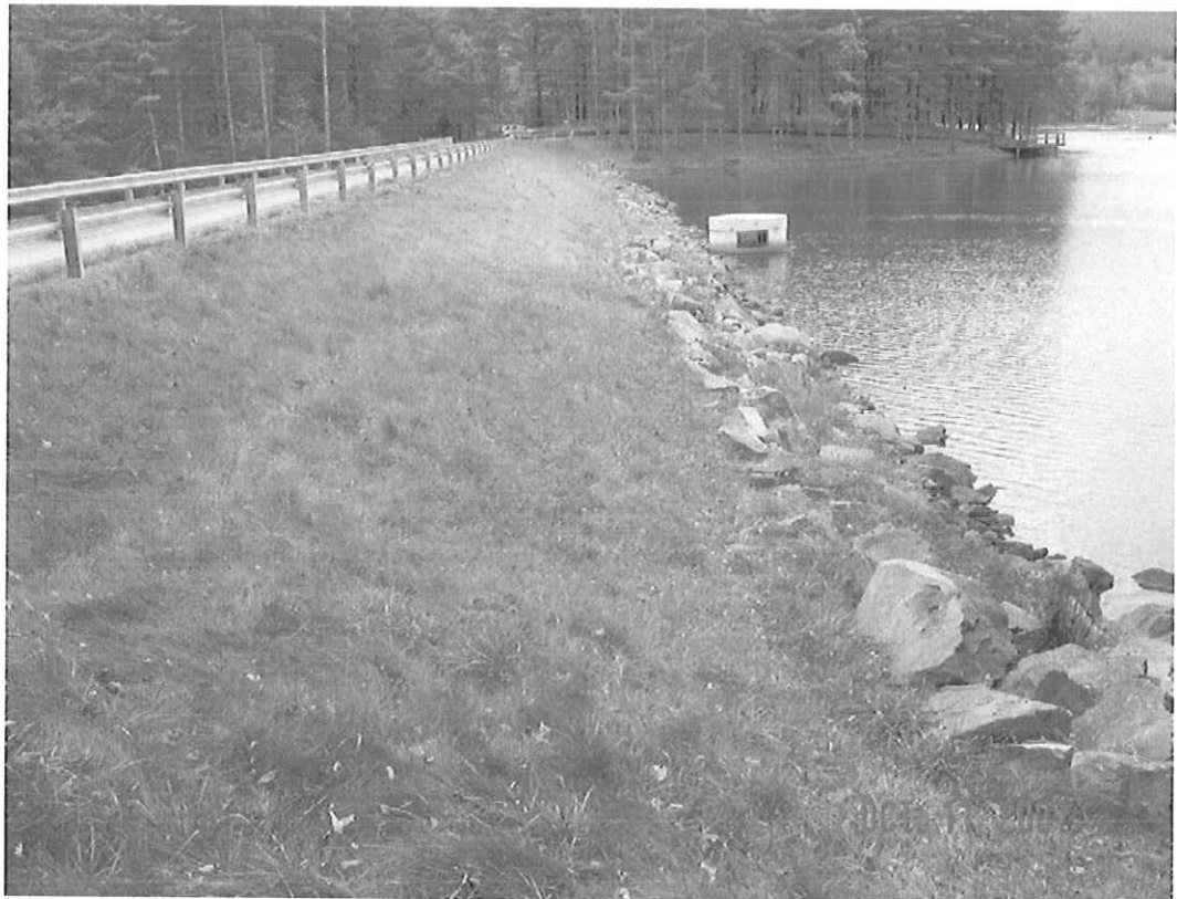
MONCOVE DAM MODIFICATION, MONROE CO., WV
