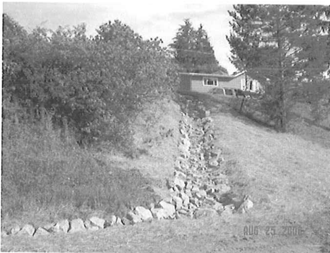
Erosion Repair – Rip Rap Armored Ditch
