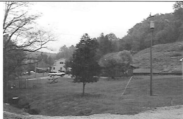
SAULS RUN STRIP AND LANDSLIDE AML related slip threatening residences along Sauls Run
