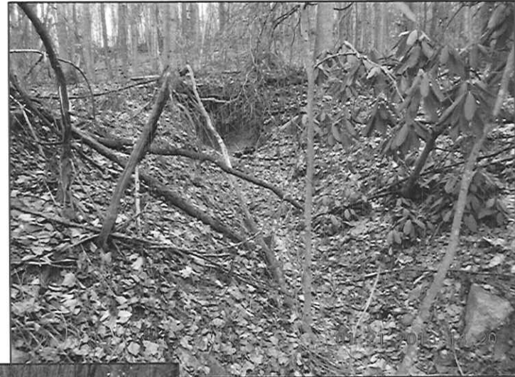
Photo E – Collapsed Portal Area
