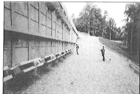
Finished wall with anchors
