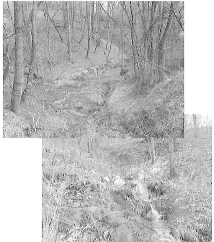
The pictures above were taken at the project site of the WV DEP's Grafton Refuse #4 and Highwall Design in Taylor County, WV.
