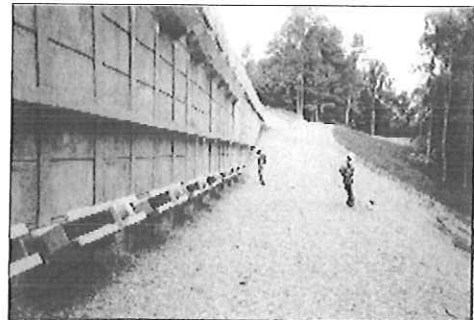
Finished wall with anchors
