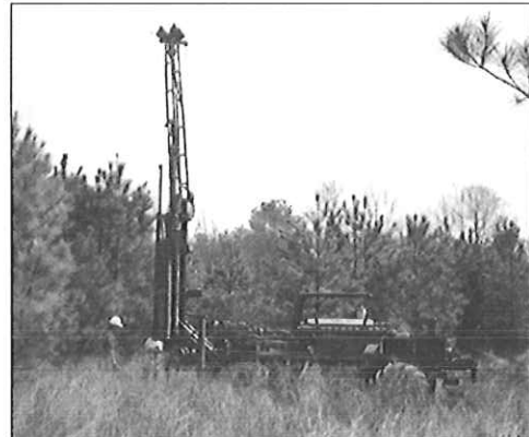
CTL's ATV can drill in rough terrain
