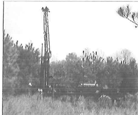
CTL's ATV can drill in rough terrain
