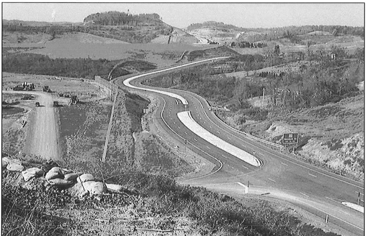
ROUTE 279, NORTH BRIDGEPORT BYPASS – COMPLETED IN 2000
