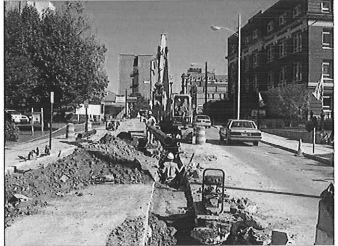
Main Street Waterline Replacement Project New 12" Ductile Iron Pipe Installation
