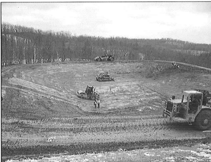
Frac pit site preparation, Ritchie County, WV
