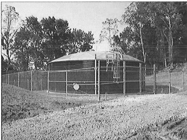
Total Project Cost = $810,000 New 250,000 Gallon Storage Tank
