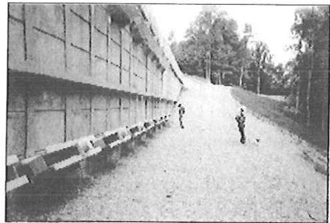
Finished wall with anchors
