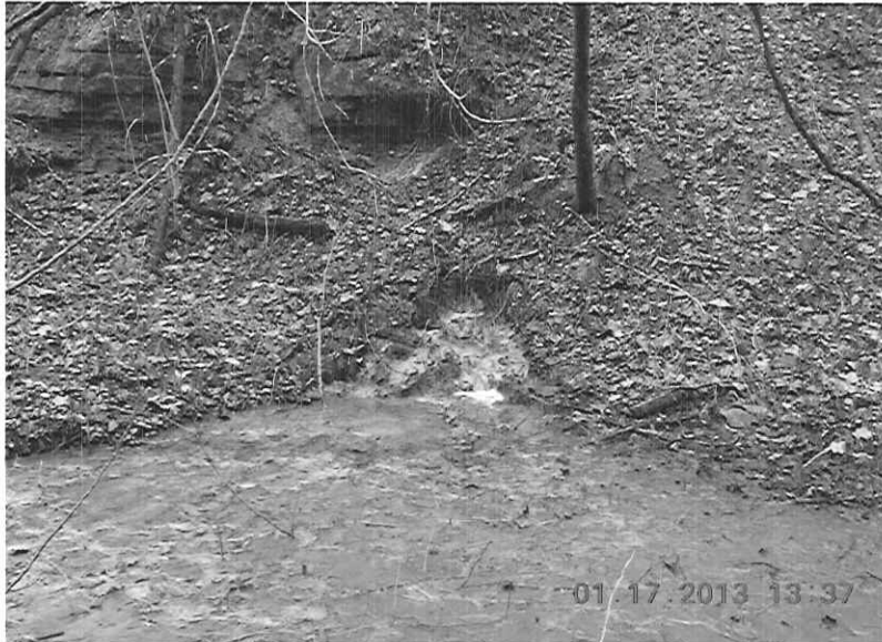
Photo "A" – Pepper Portal Mine Drainage
