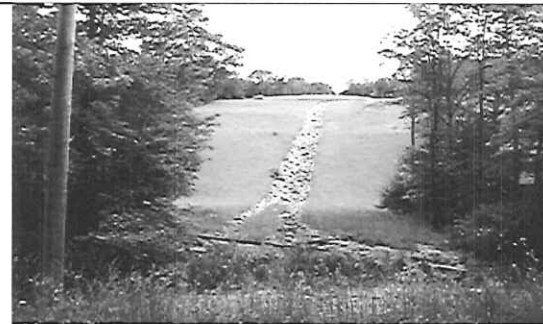
Stabilized Refuse Pile MUDDY CREEK TIPPLE COMPLEX - near Mt. Storm, Grant County, WV
