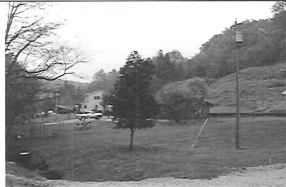
SAULS RUN STRIP AND LANDSLIDE AML related slip threatening residences along Sauls Run
