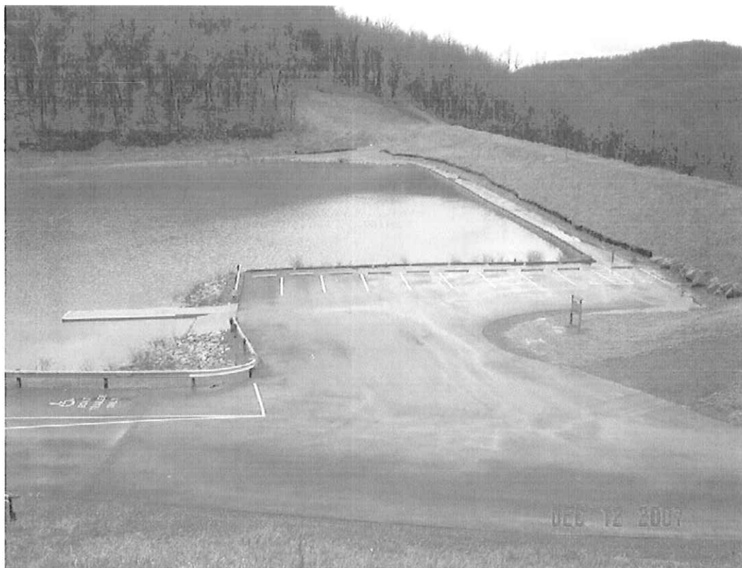
BAILEY DAM MODIFICATION, MONONGALIA CO., WV
