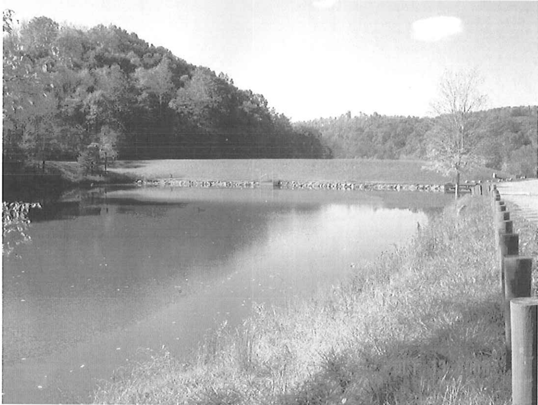
JIMMY LEWIS DAM MODIFICATION, MERCER CO., WV
