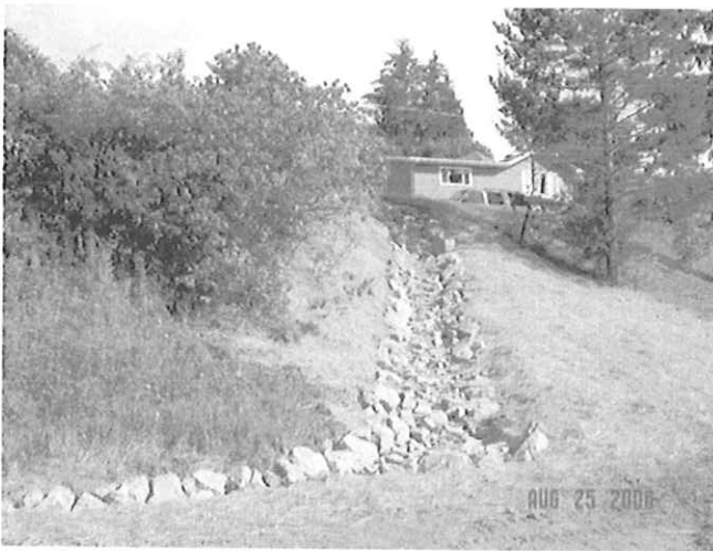
Erosion Repair – Rip Rap Armored Ditch
