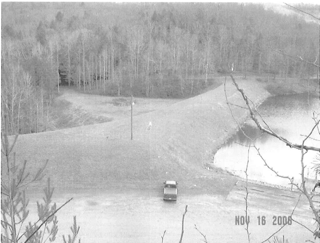
PLUM ORCHARD DAM MODIFICATION, FAYETTE CO., WV
