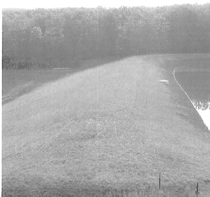
WILSON DAM MODIFICATION, HAMPSHIRE CO., WV
