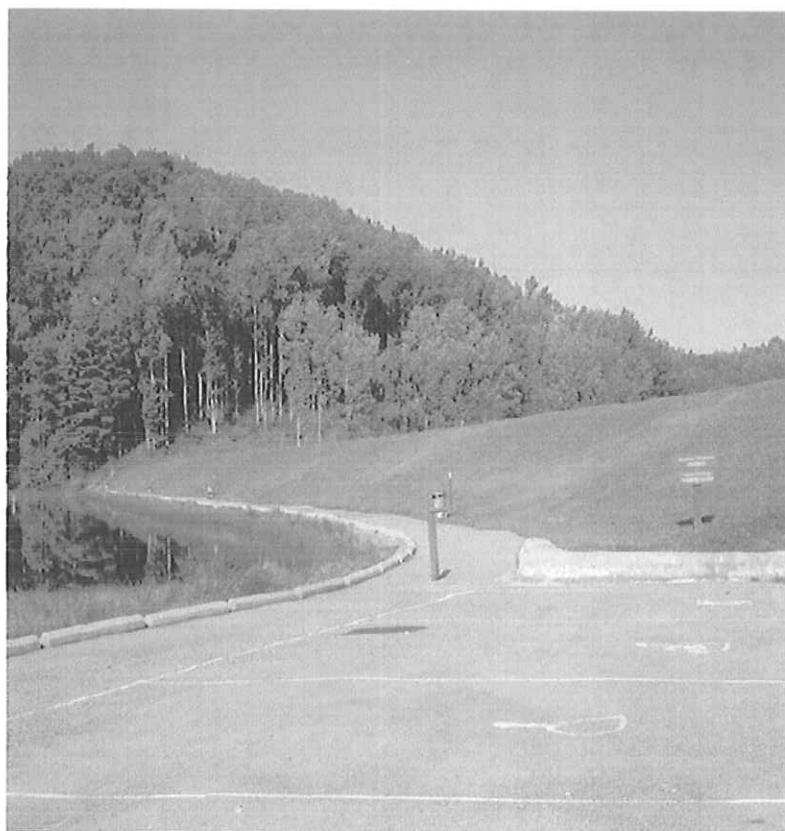
TETER CREEK DAM MODIFICATION, BARBOUR CO., WV
