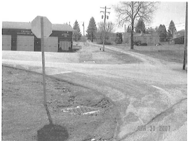
New Storm Drains and Catch Basins
