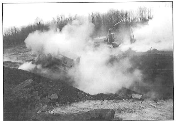
Jamison Burning Refuse Reclamation Project
