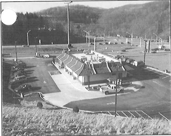
CTL Engineering, Inc. provided surveying services for this McDonald's site in Star City, West Virginia
