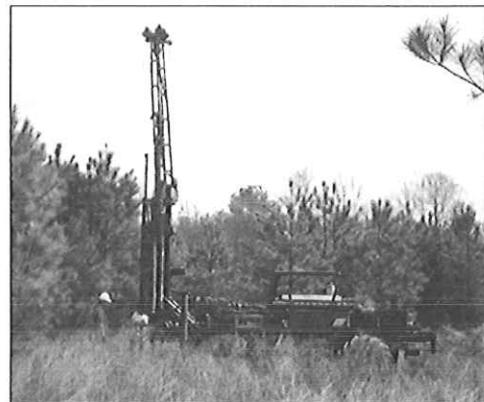
CTL's ATV can drill in rough terrain
