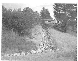
Erosion Repair - Rip Rap Armored Ditch
