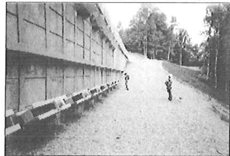
Finished wall with anchors
