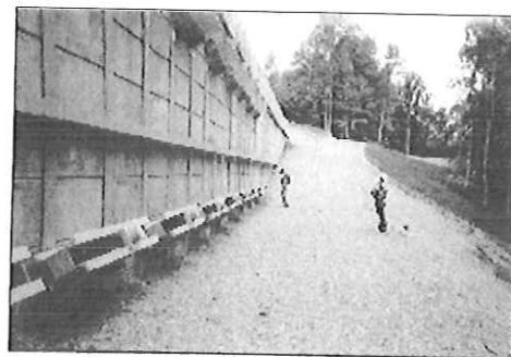
Finished wall with anchors
