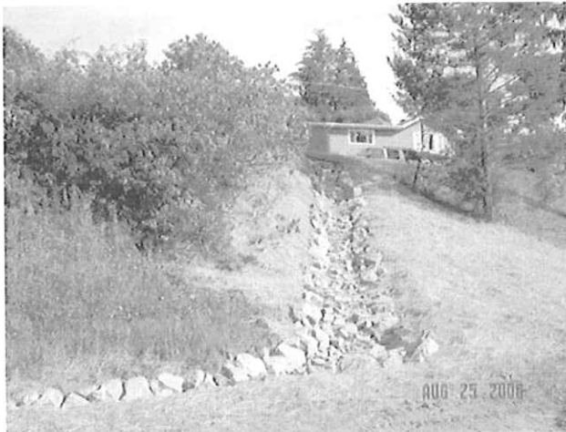
Erosion Repair – Rip Rap Armored Ditch
