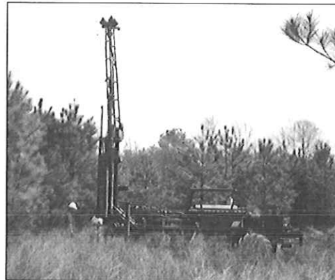
CTL's ATV can drill in rough terrain
