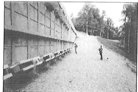
Finished wall with anchors
