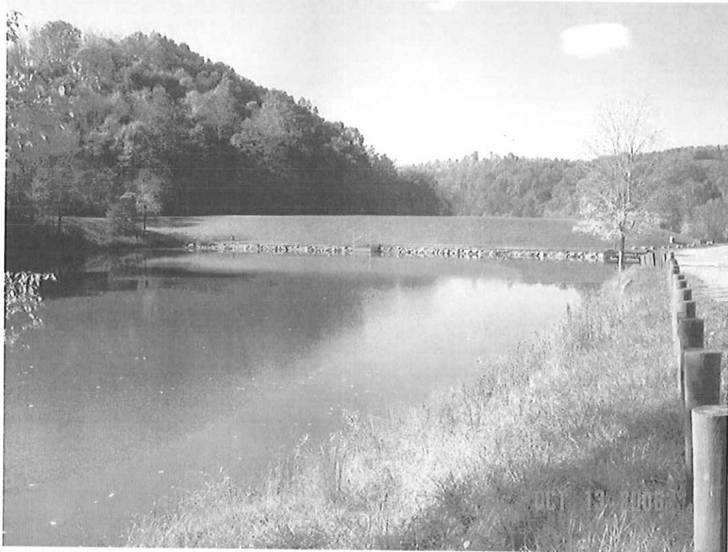
JIMMY LEWIS DAM MODIFICATION, MERCER CO., WV
