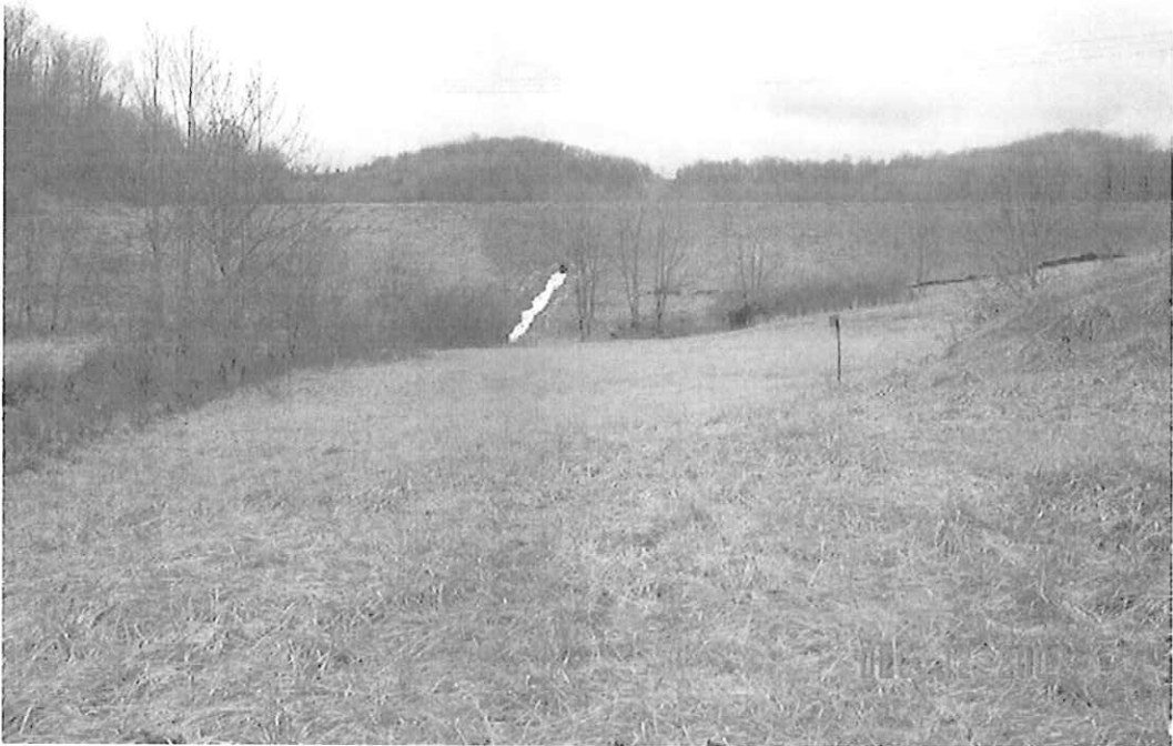
LEMLEY DAM MODIFICATION, MONONGALIA CO., WV
