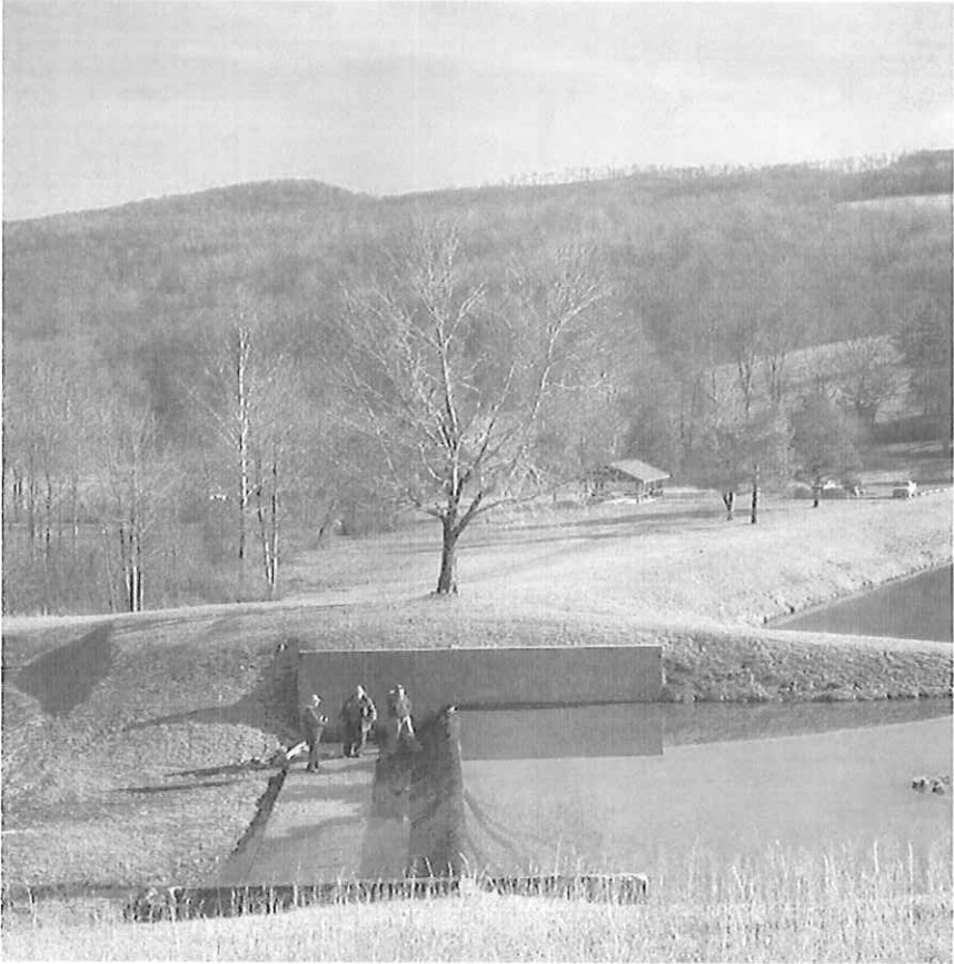
BELINGTON DAM MODIFICATION, BELINGTON, WV
