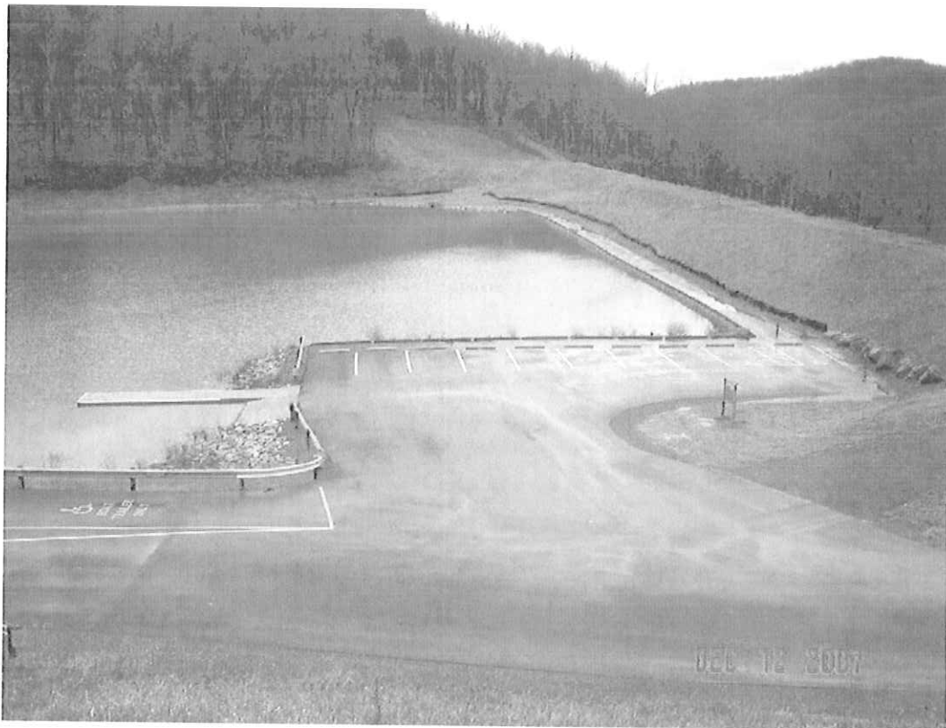
BAILEY DAM MODIFICATION, MONONGALIA CO., WV
