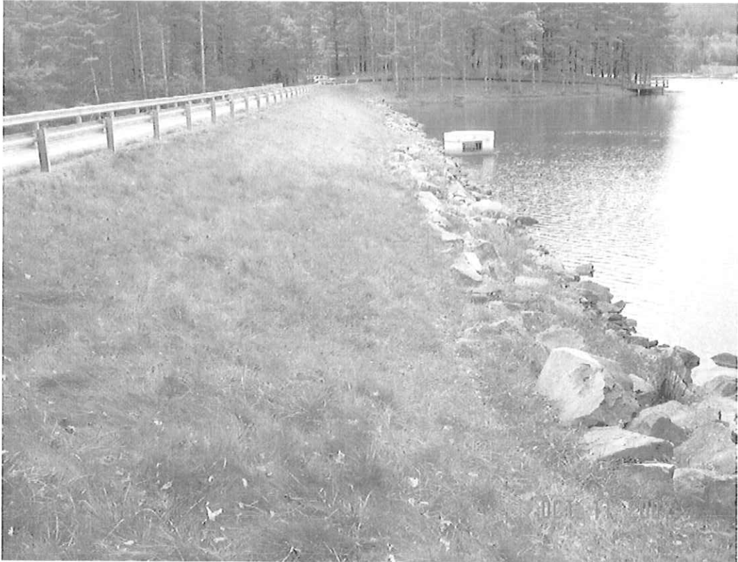
MONCOVE DAM MODIFICATION, MONROE CO., WV
