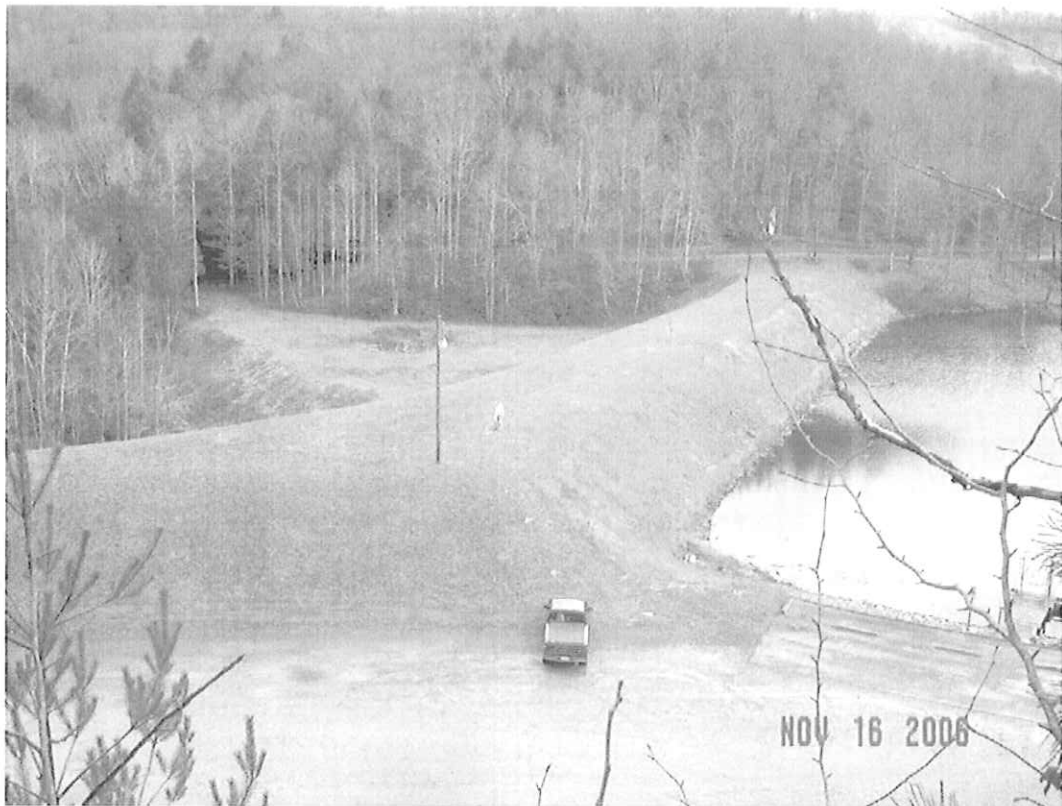
PLUM ORCHARD DAM MODIFICATION, FAYETTE CO., WV
