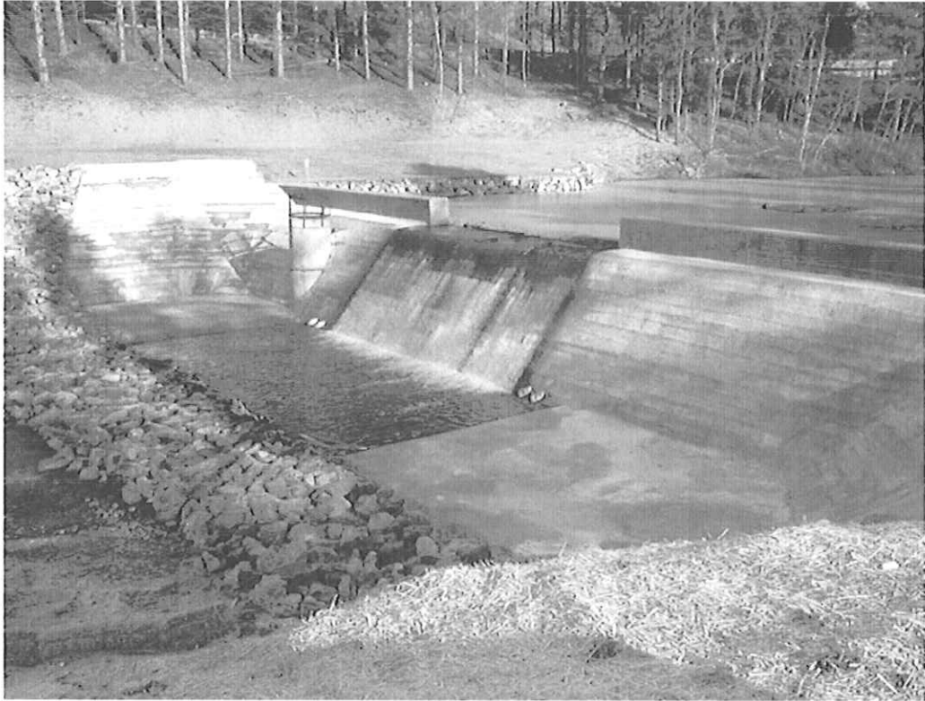
THOMAS DAM MODIFICATION, THOMAS, WV
