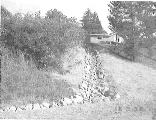
Erosion Repair – Rip Rap Armored Ditch
