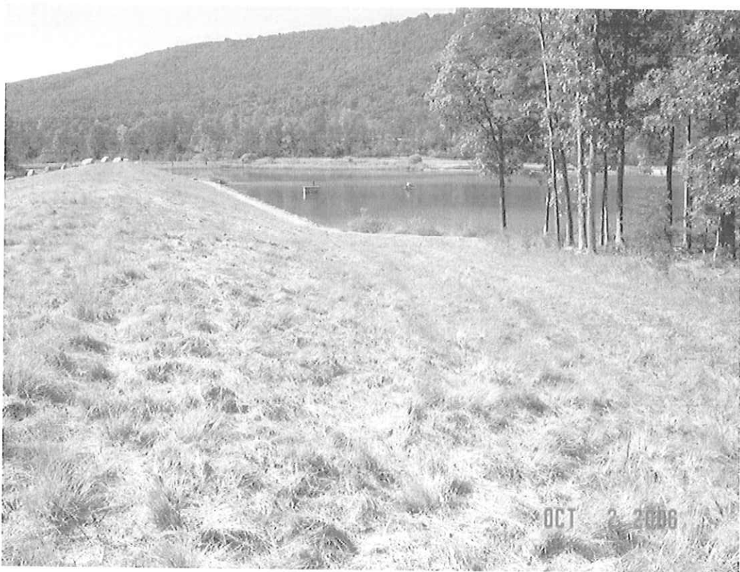
WARDEN LAKE DAM MODIFICATION, HARDY CO., WV
