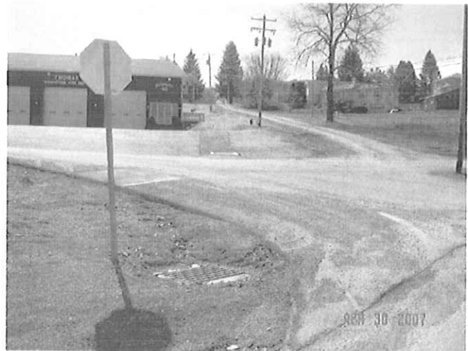
New Storm Drains and Catch Basins
