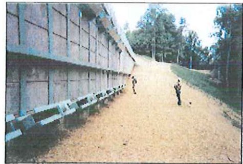
Finished wall with anchors
