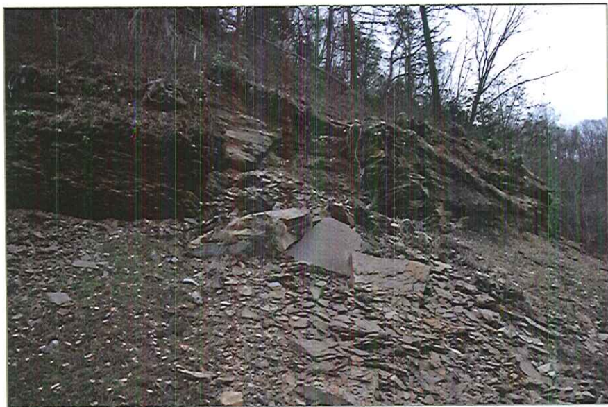
Photo E - Landslide
