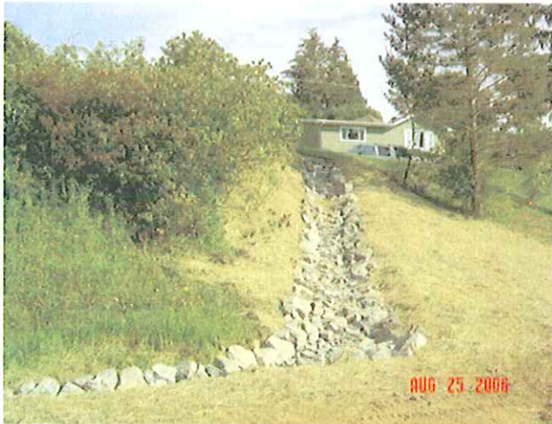
Erosion Repair – Rip Rap Armored Ditch
