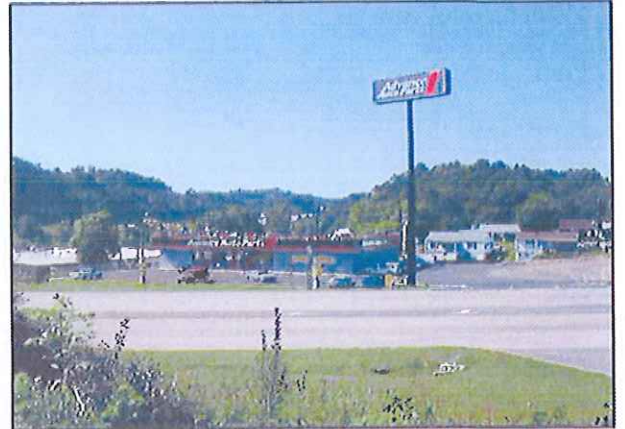
CTL Engineering of West Virginia, Inc. provided site plans for this Advance Auto Parts Store in Morgantown, West Virginia
