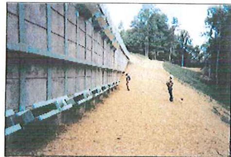
Finished wall with anchors
