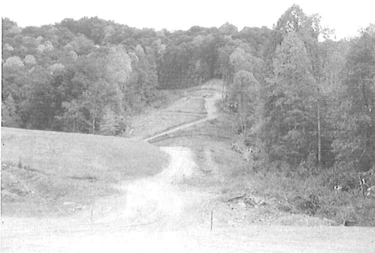
Transmission Line Construction
