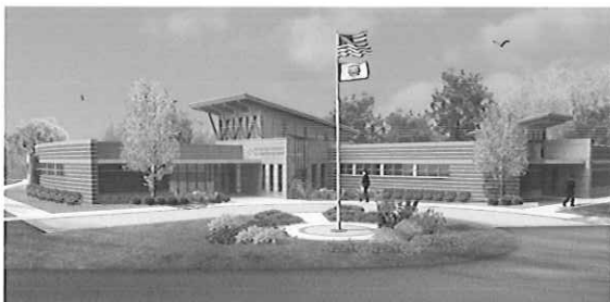
Mercer Health Center, Green Valley, WV
