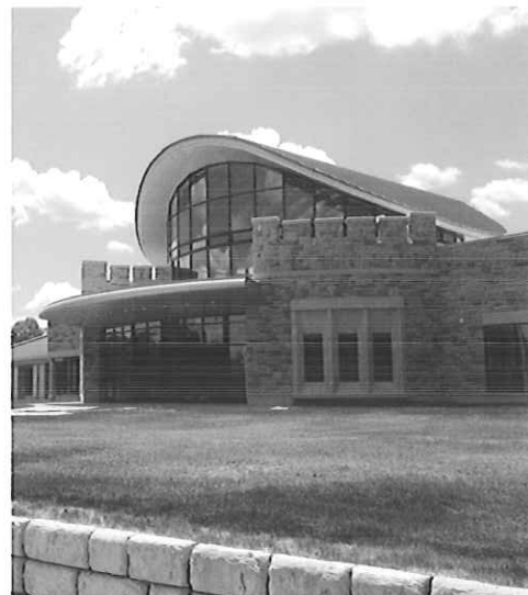
WVARNG Readiness Center - Elkins
