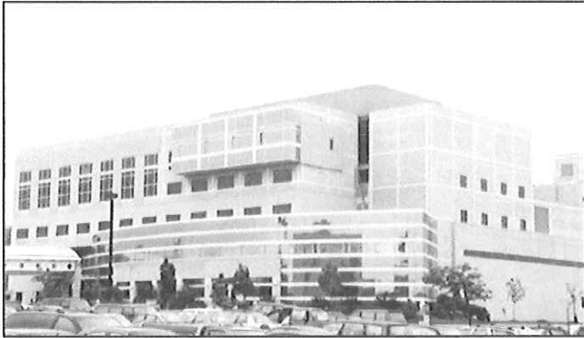
LAKE WEST HOSPITAL Willoughby, Ohio
