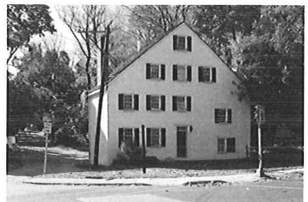
The Rowland House / Shovel Shop
